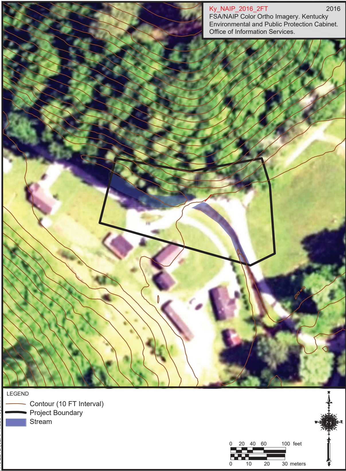
CR 1041 bridge (007C00003N) over York Branch (Item No. 11-10002.00) in Bell County, Kentucky.
