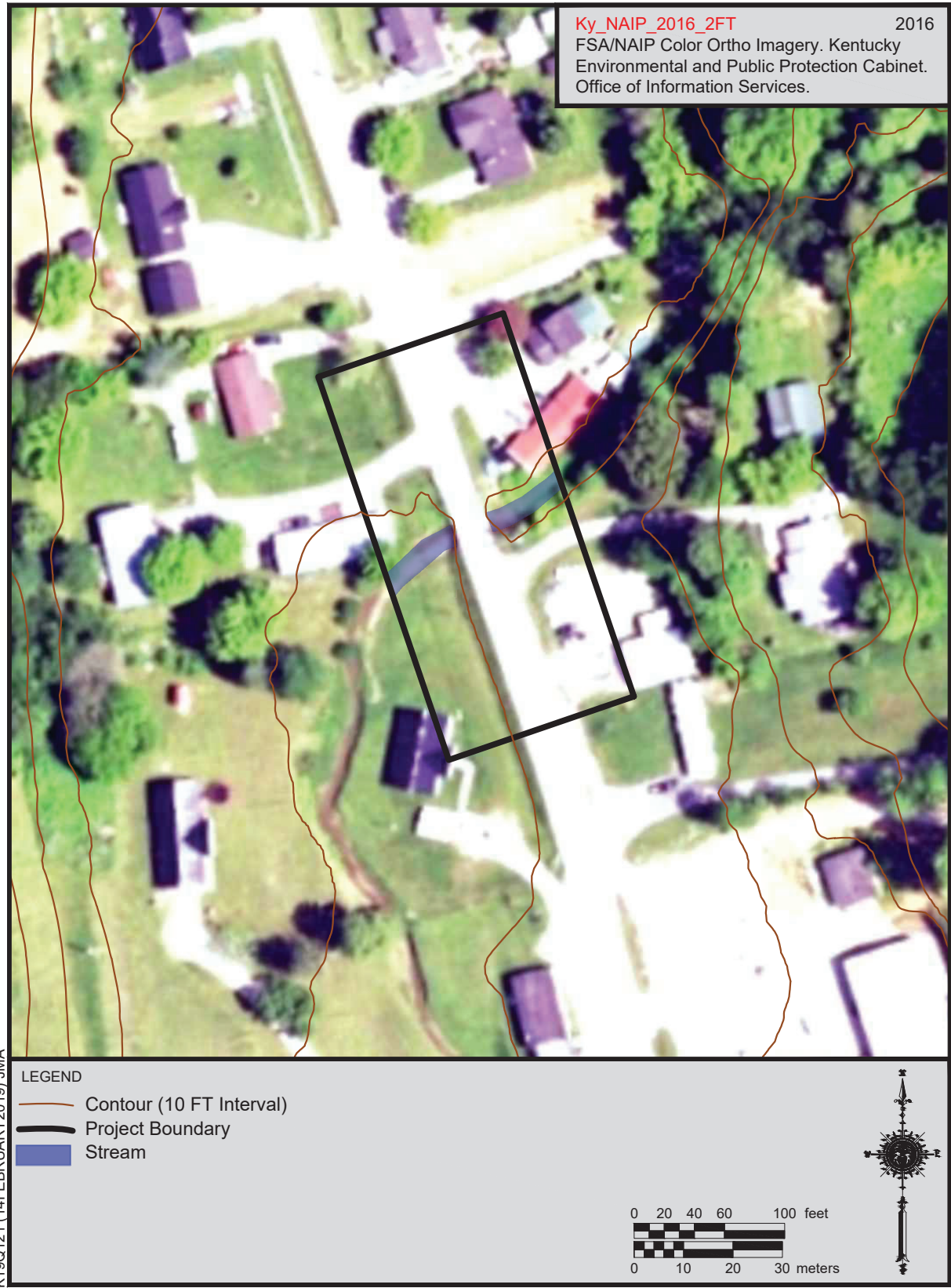
US 421 bridge (026B00002N) over Island Creek Branch (Item No. 11-10039.00) in Clay County.
